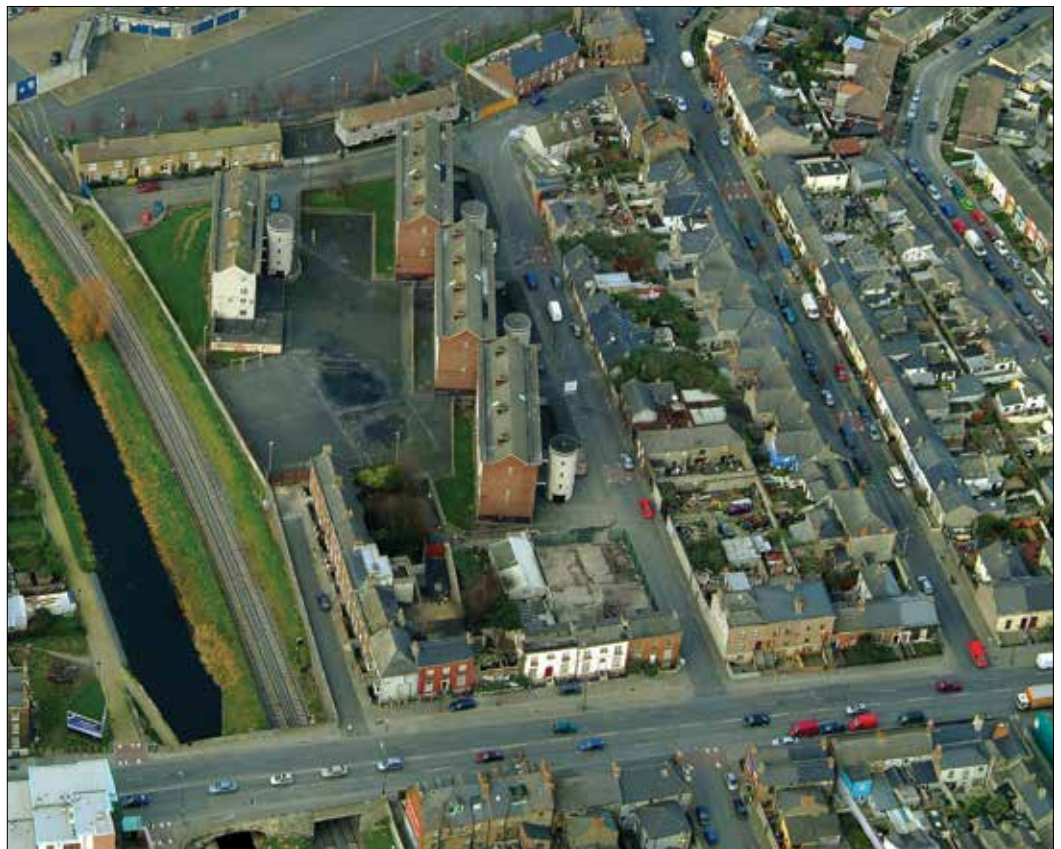
Croke Villas and Environs: Phase one of seven units under construction on Ballybough Road, 76 units at planning stage, completion expected in 2019.
