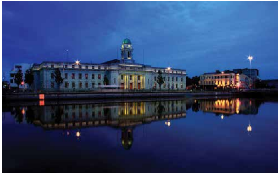
Cork City Council HQ at City Hall on Anglesea Street.
