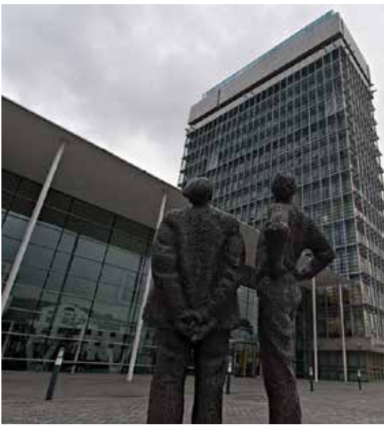
Cork County Council HQ at County Hall on Carrigrohane Road.
