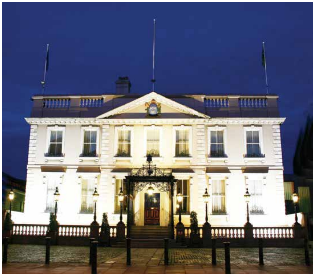
Dublin's Mansion House on Dawson Street – the residence for the city's Lord Mayor.
