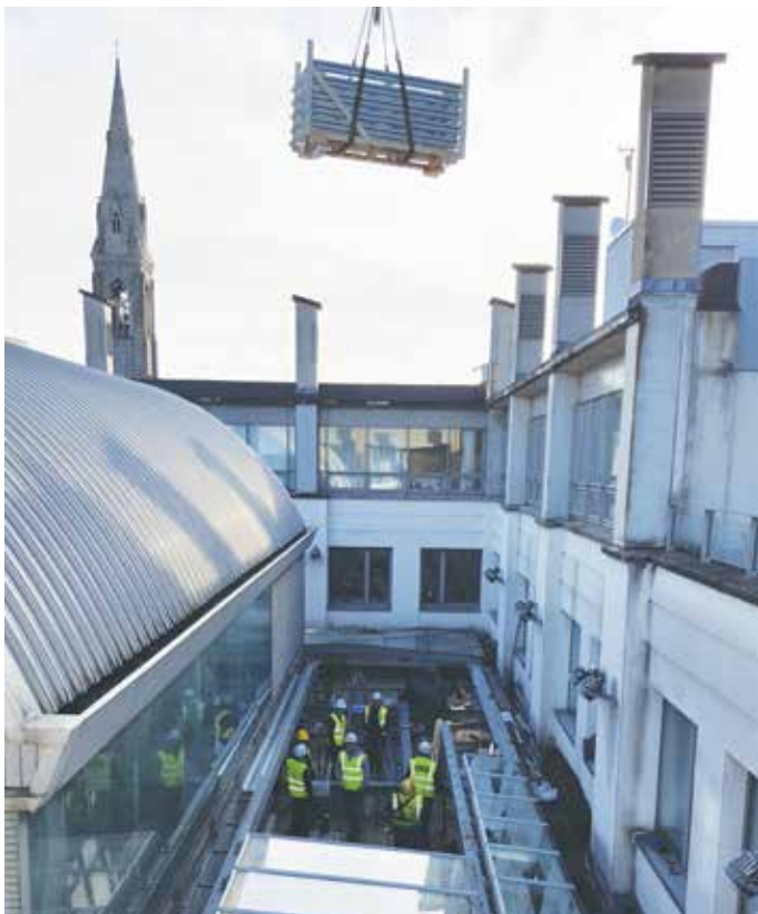
Installation of new roof glazing system from Velux.
