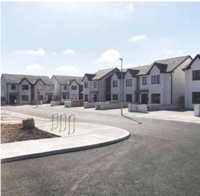
The 18 new social housing units in Rathangan comprise of one, two, three and four-bedroomed A-rated properties.
