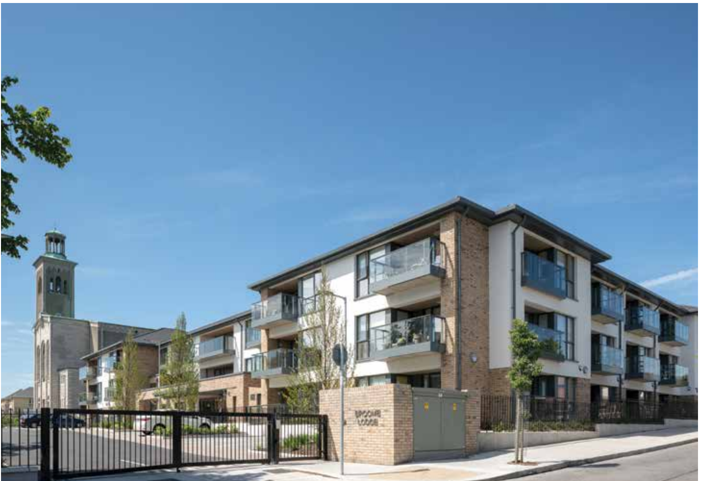
Broome Lodge in Cabra (one of over 20 schemes in operation by Clann across the country) was designed following the principles of Universal Design and has received plaudits for its design, comfort and place in the heart of the Dublin 7 community.
