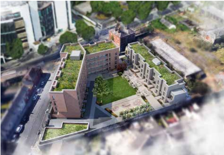
DCC's Housing Team is piloting BIM on several projects with multiple benefits being generated.
