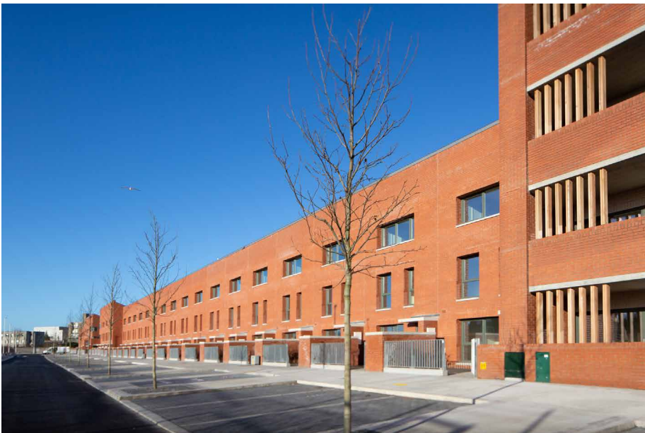
Dublin City Council's social housing development on Margaret Kennedy Road, Dublin 8.
