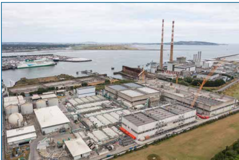
An aerial view of the Ringsend Wastewater Treatment Plant Upgrade Works.
