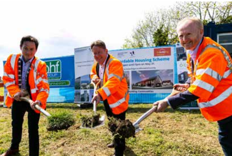
Fingal County Council’s Affordable Housing Scheme at Dun Emer in Lusk took a major step forward in May 2021 when the first sod was turned on the construction site. Pictured (l-r): Deputy Mayor of Fingal, Cllr Robert O’Donoghue, Minister for Housing, Local Government and Heritage, Darragh O’Brien TD, and Mayor of Fingal, Cllr David Healy.
